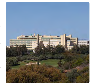
Hospital Costa del Sol
